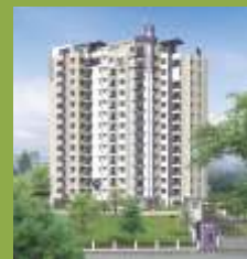
Crescent Kings Spear Mini Bypass Road, Calicut
